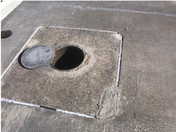
Photo #7: Overflow skimmer location.
