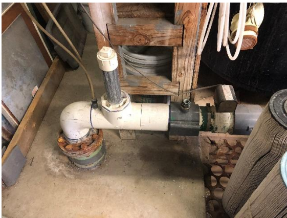
Photo #15: Chlorine and CO2 injection points
