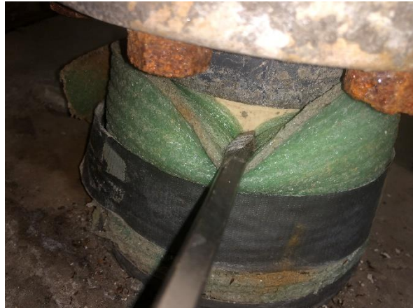
Photo #10: Further detail of Photo #9.
