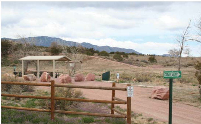
Existing Spring Creek Park
