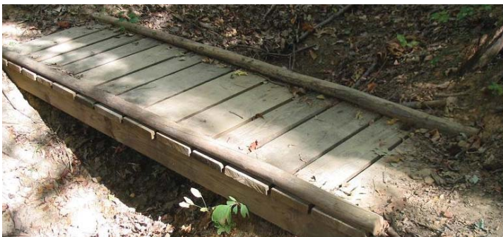
Example Of A Timber Bridge
