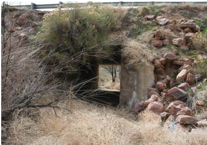
Existing Box Culvert At Hwy 115
