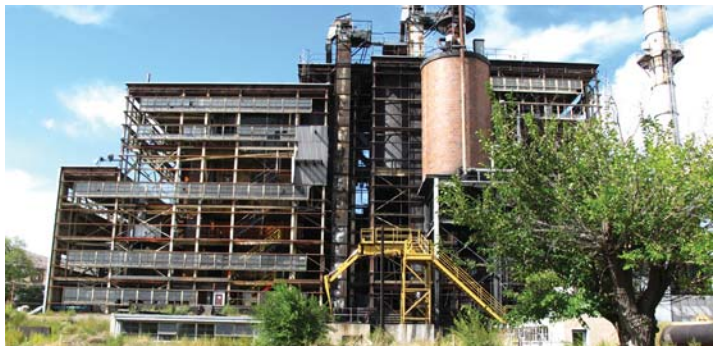
WN Clark Power Plant
