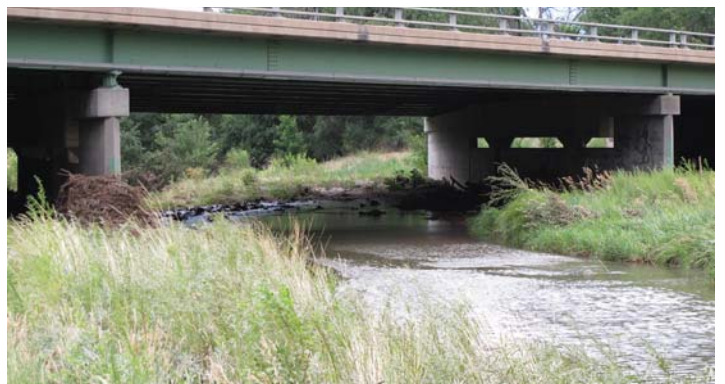
View Of Hwy 50 Underpass
