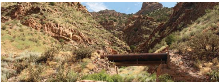
View North Of Tunnel Drive Towards Fremont Peak
