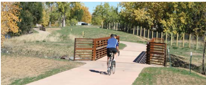
Prefabricated Bridge Along Multi-Use Trail
