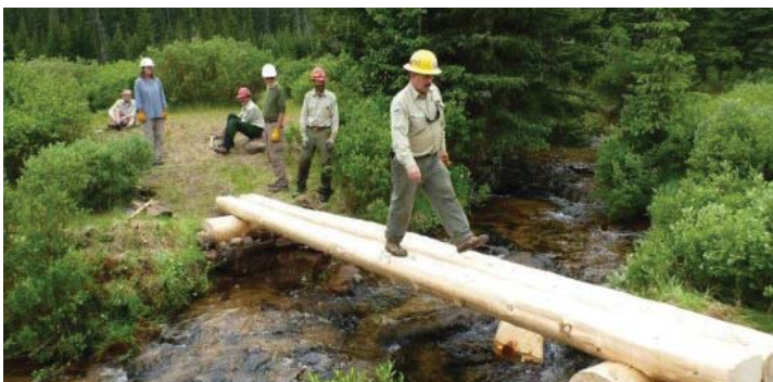
Example Of A Narrow Bridge On A Single Track Trail
